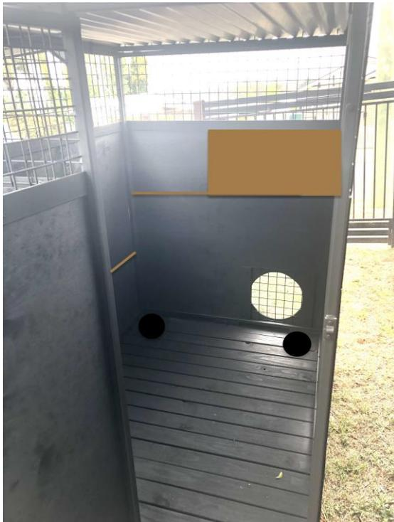
**Figure 1:** Inside view of prototype Vennel showing roof, ventilation mesh at the top of the wall, shelf and nest box, hole in the wall where the Tasmanian devil PVC pipe trap would be attached on the outside, and holes in the wooden floor for removal of faeces. This design has been modified, and the Vennel is bigger with an insulated overhanging roof and walls made from insulation panels used for cool rooms.
